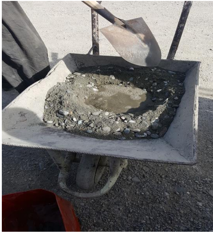
Figure 1. Mixing of the concrete ingredients
